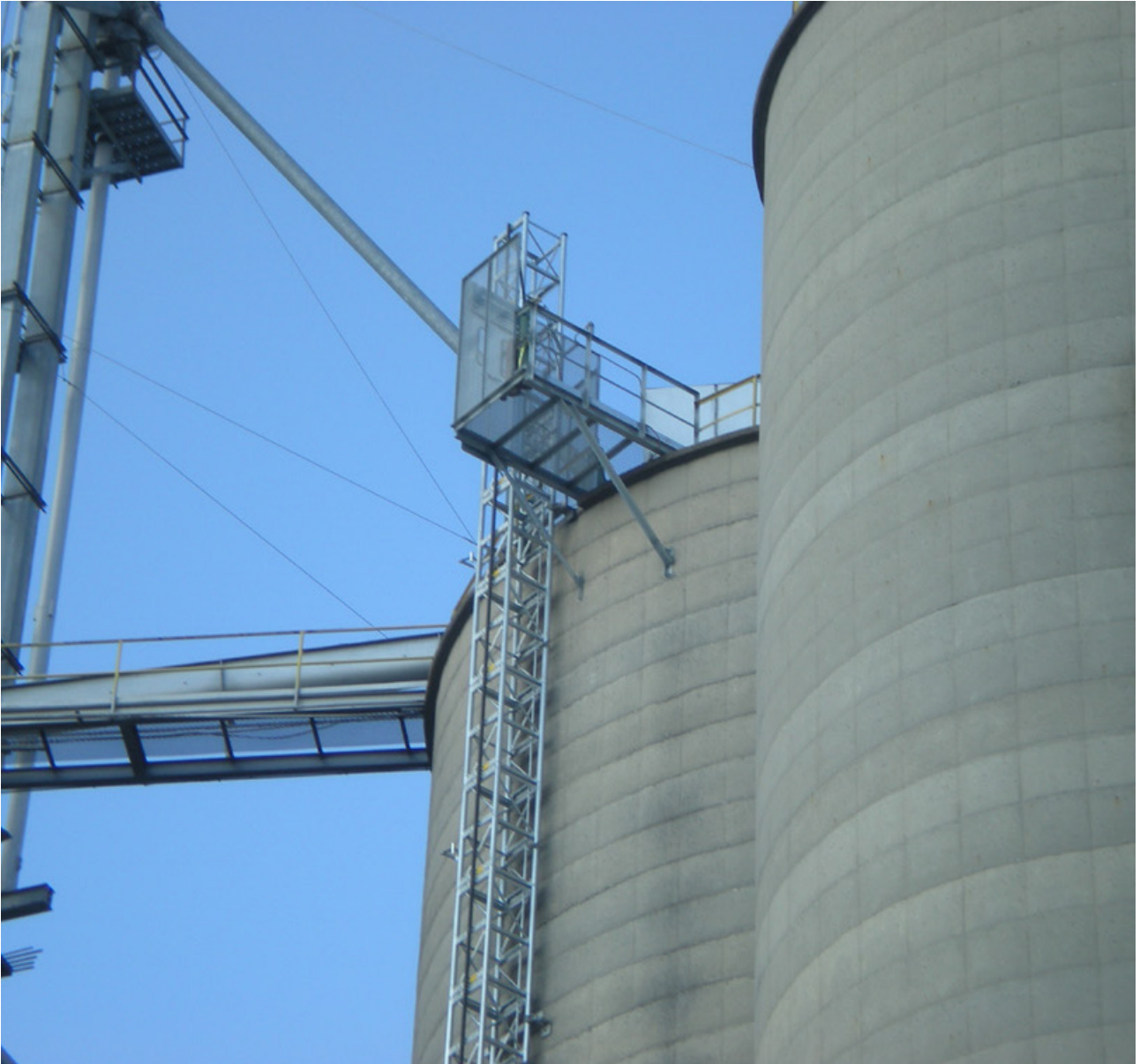
Graincorp Grain Handling Facility, QLD, Australia
