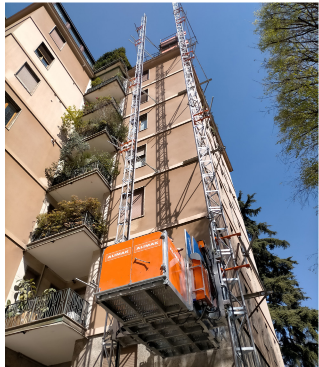
Penthouse Renovation, Milano, Italy
