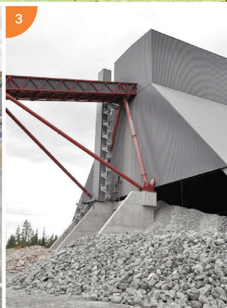
Ore stockpile Elevator: ALIMAK SE 1000 Capacity: 1000 kg Lifting height: 48 m
