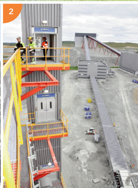
Surface Crusher Elevator: ALIMAK SE 1000 Capacity: 1000 kg Lifting height: 24 m
