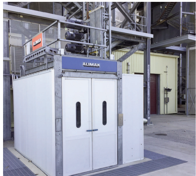
The large capacity Alimak rack and pinion elevator ensures easy access to the scrubber at any moment.
