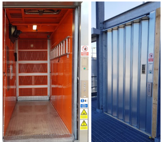
Data Centre, Slough, United Kingdom
