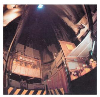
for a 90 second load/unload cycle, the combined travelling distance of the three hoists were conservatively estimated at 65,000 km's each year – well in excess of the usual maximum travelling distance of construction hoist equipment.
