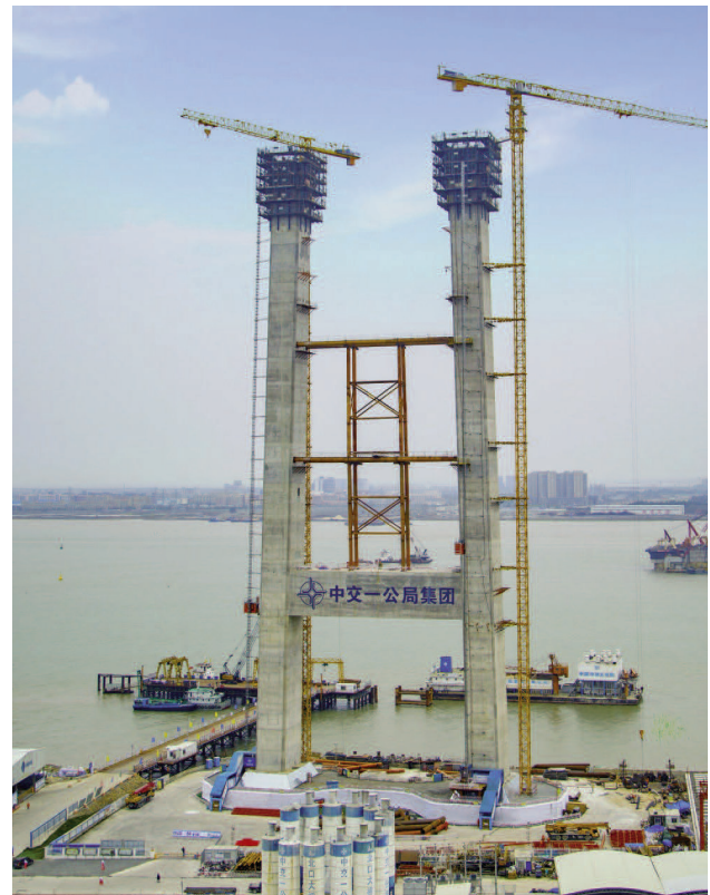
Two Alimak hoists service the construction of a new double-deck suspension bridge in China
