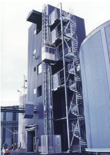
The green liquor filter building.
