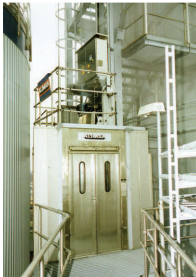
The 1200-kg capacity ALIMAK SE-12 waits at a bleach tower landing.
