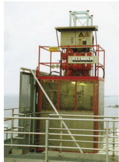
The top landing of one of the bleach towers.
